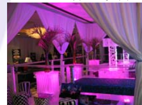
Full venue lighting—LED Wash lights
